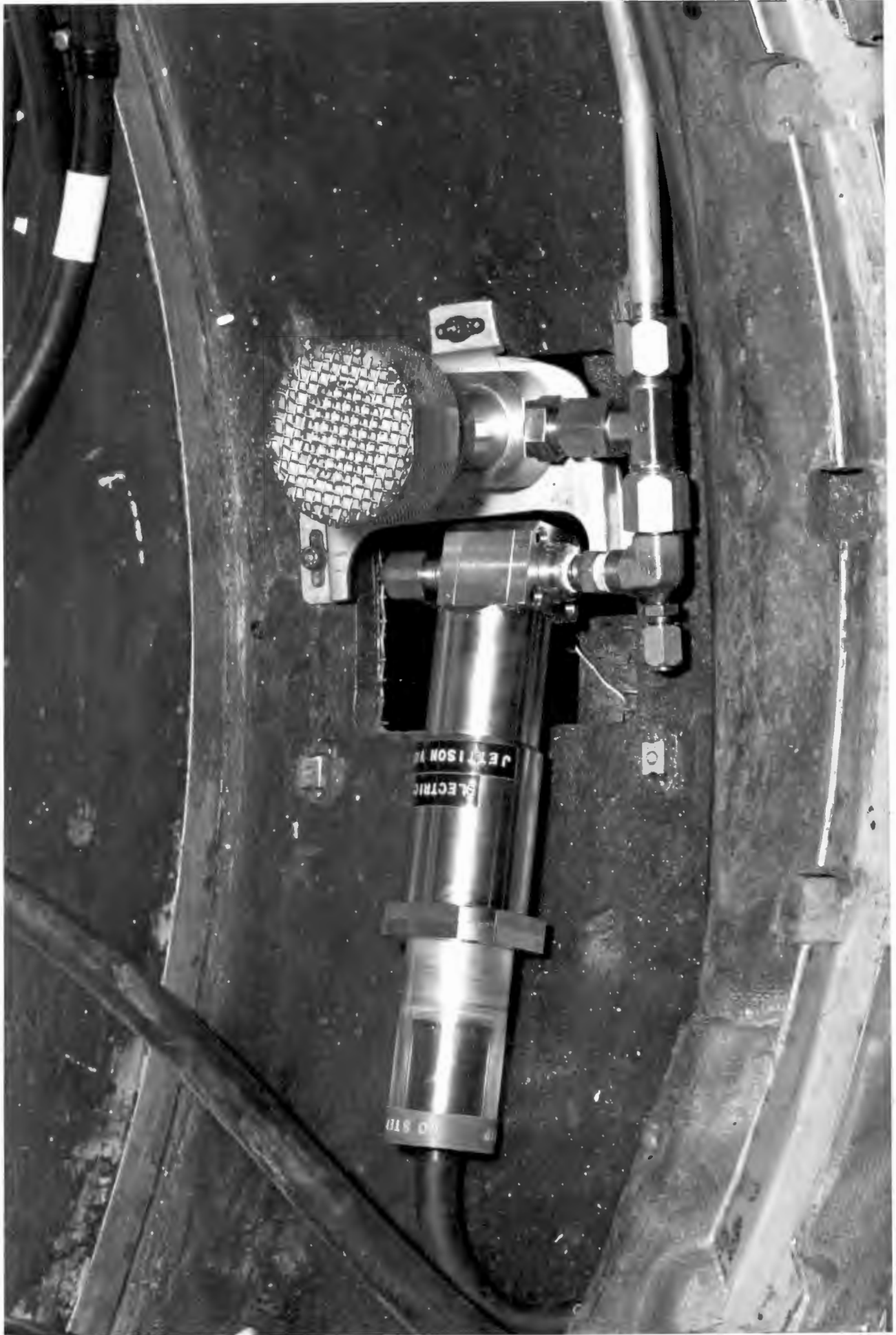
AFT JETTISON VALVE INSTALLATION
