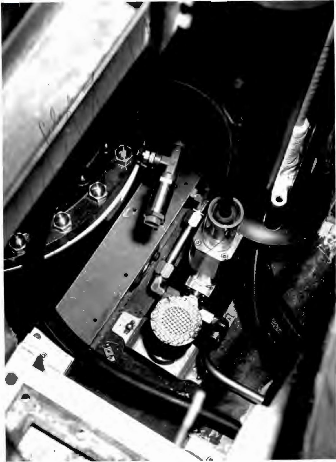
FORWARD JETTISON VALVE INSTALLATION
